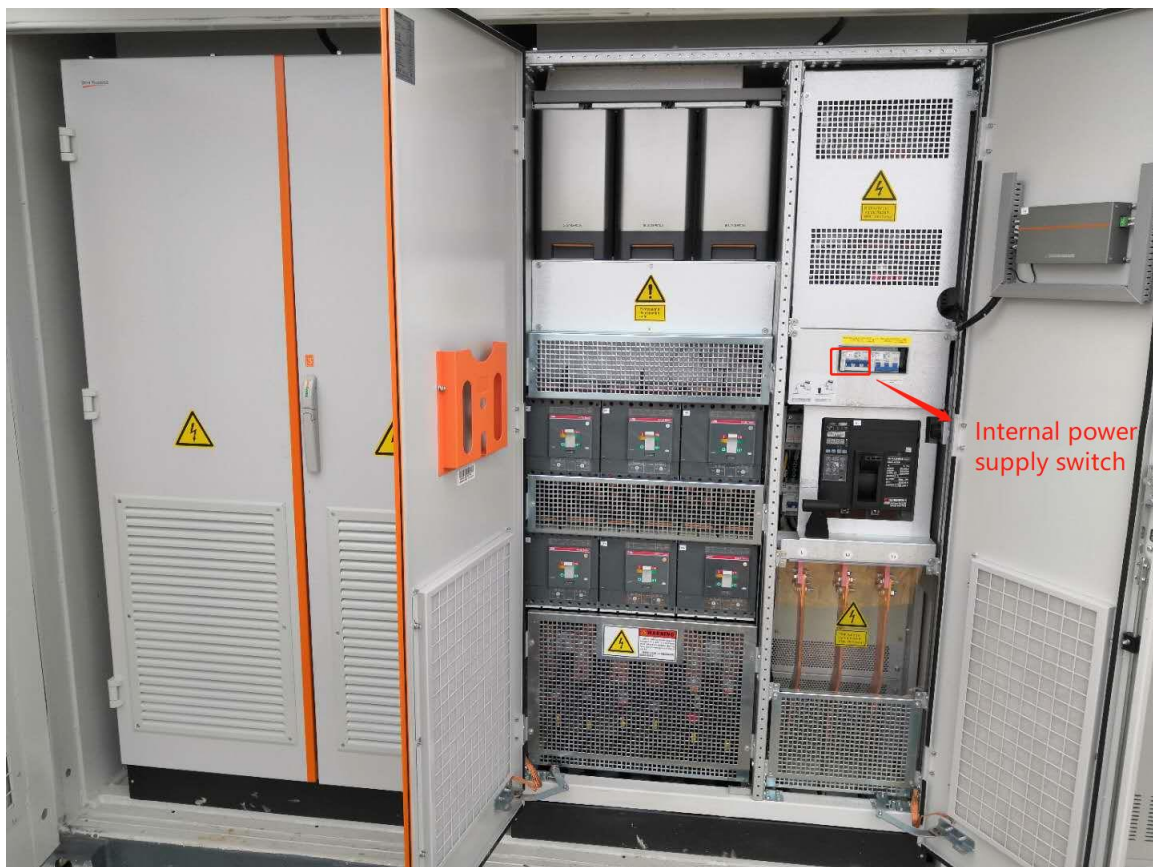
Figure 7: Internal power supply switch
